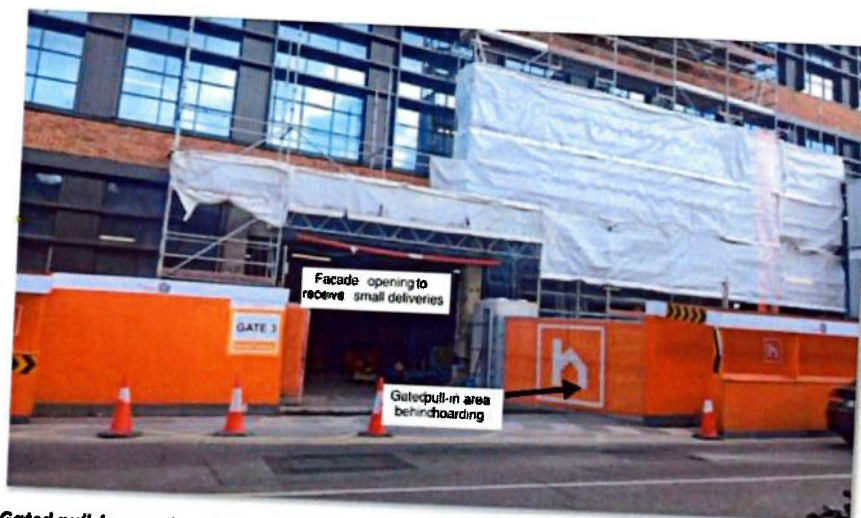
Gated pull-in area for off-loading deliveries using a tower crane – recent city centre project
