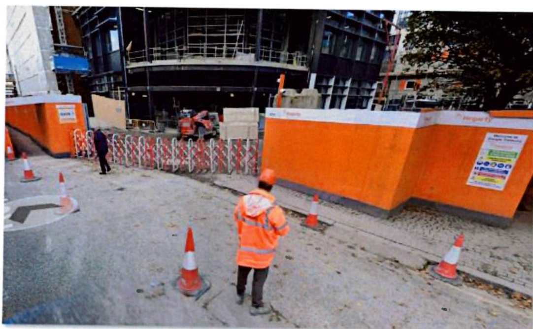
Pull-in Area for Deliveries – Controlled by Traffic Marshal
